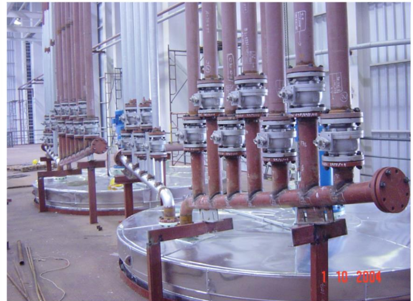
PIPING AROUND BATCH BLENDER TANK TANK INSTALLATION PROJECT FOR APOLLO (THAILAND) CO., LTD.
