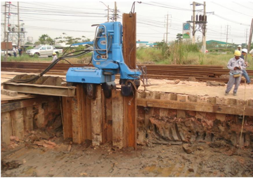
INTER LOCK SHEET PILE AND STEEL BRACING FOR TIE IN PIT
