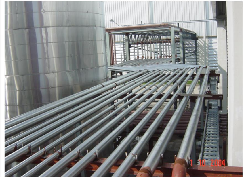
PIPING ARRANGEMENT ON BRIDGE AND RACK TANK INSTALLATION PROJECT FOR APOLLO (THAILAND) CO., LTD.
