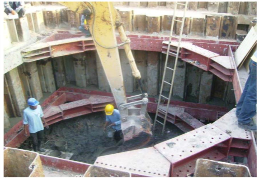
INTER LOCK SHEET PILE AND STEEL BRACING FOR TIE IN PIT
